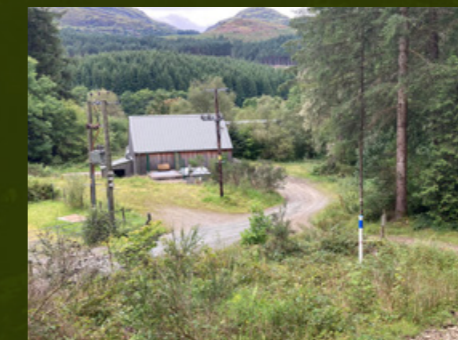
Inveronich hydro electric turbine house. The blue and white pole marks the position of the pipeline.
