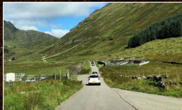
The straight section of the old military road is to be doubled in width to form a construction "relief road", but traffic lights will be required at the hairpins.
