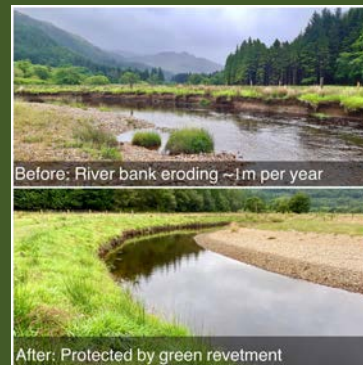
After: Protected by green revetment
