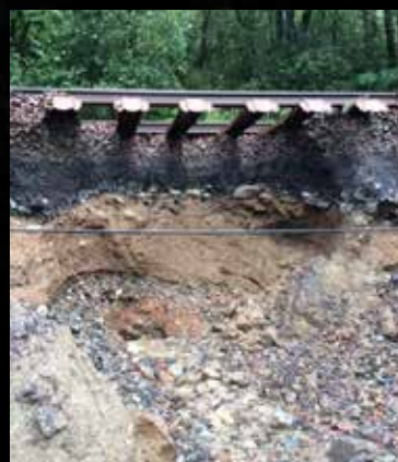
Floodwater from the same event seriously damaged the West Highland railway track in Strathfillan
